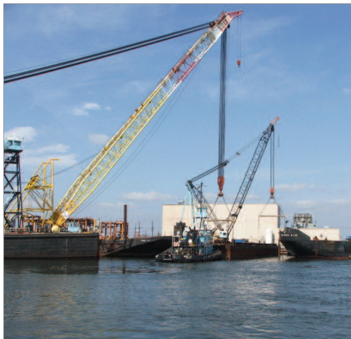
Contaminated dredge spoils are loaded into one of Donjon's derrick barges.
